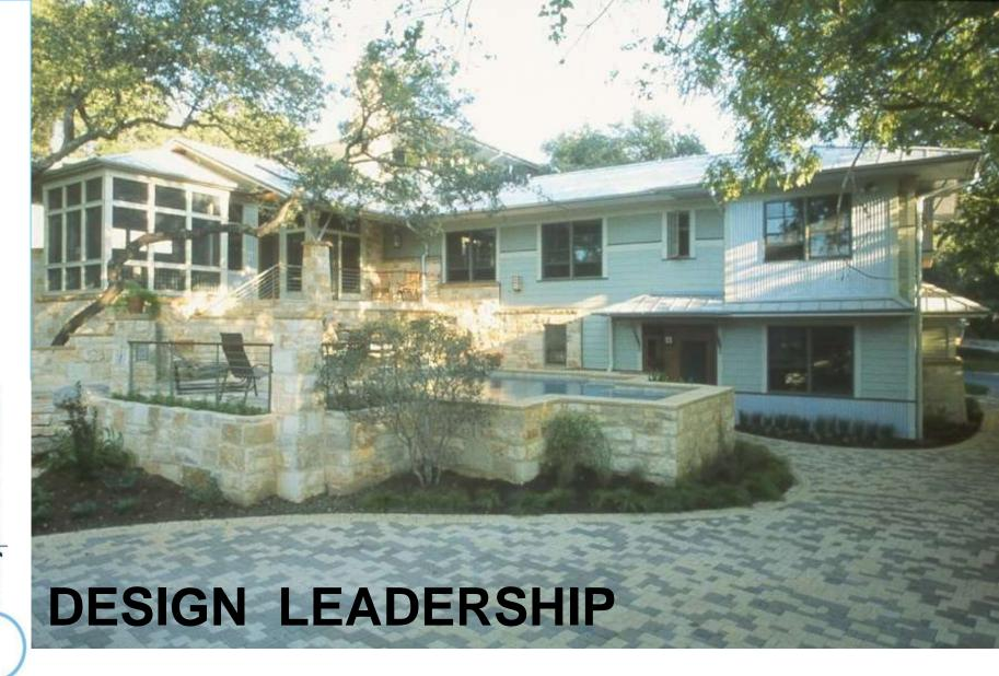
Window shading – the DESIGN of the roof overhangs with regard to the windows - saves more energy than \$16,000 solar collectors.
