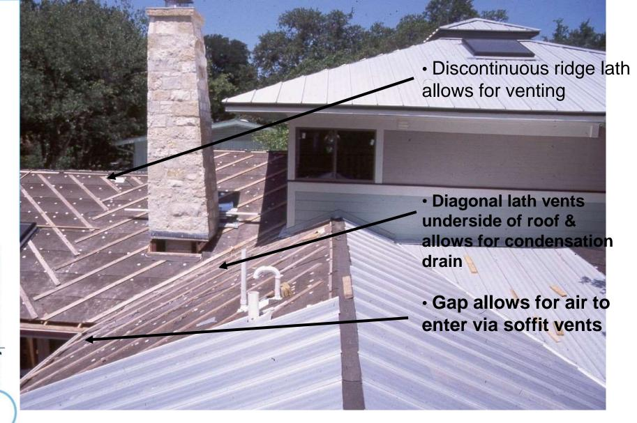
The Barley|Pfeiffer Floating Radiant Barrier Roof System Galvalume roofing installed with a vented airspace beneath.
