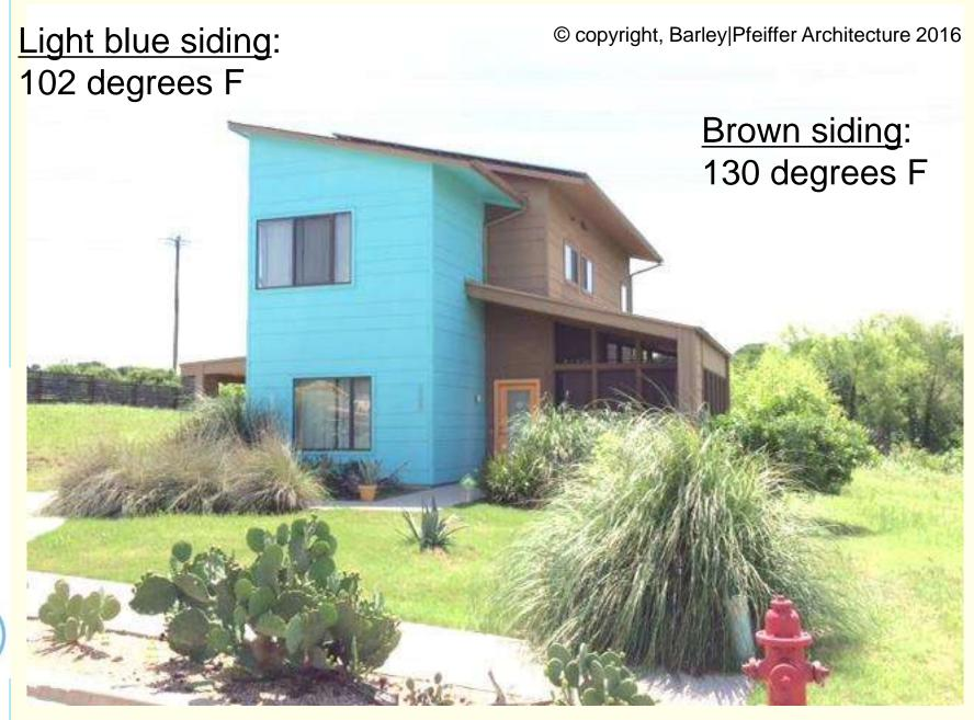
The effect of radiant heat gain on conductive "R" value
